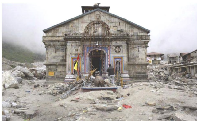
Figure 7. Thick depositions (1–1.5 m) of poorly sorted sediments in the outwash plain; the steps of the temple are filled.
