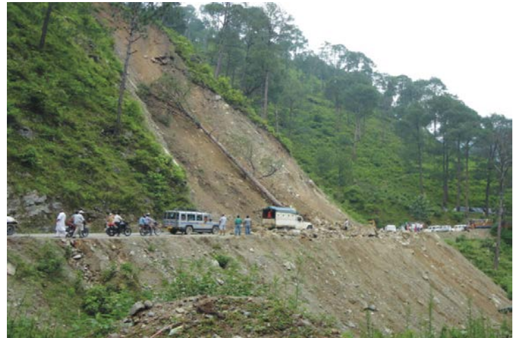
Photo 2: Landslides in Rudraprayag - Guptkashi road
