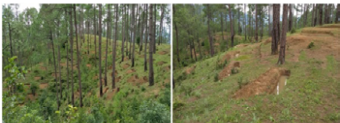
Fig. 1. Groundwater augmentation measures (contour trenches) in the catchment of experimental spring (based on spring sanctuary concept)
